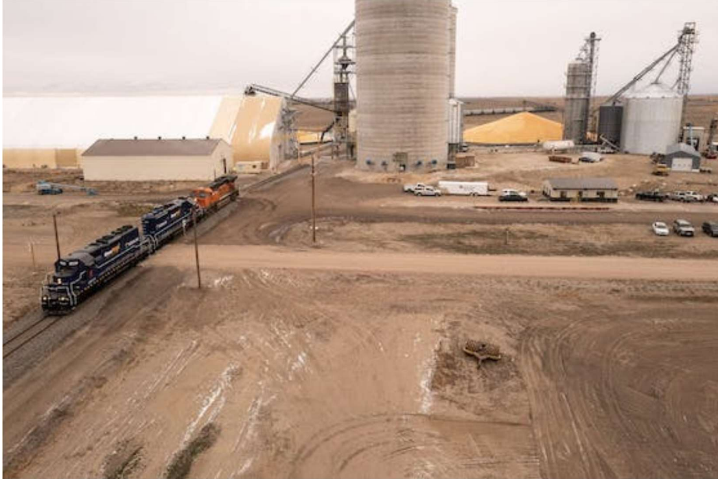
OmniTRAX 419 & 420 at Grainton Shuttle Loading Facility ribbon cutting held 11 AM on Thursday, November 17, 2022. Operation is served by Nebraska-Kansas-Colorado Railway. ©2022 Chip photo.
