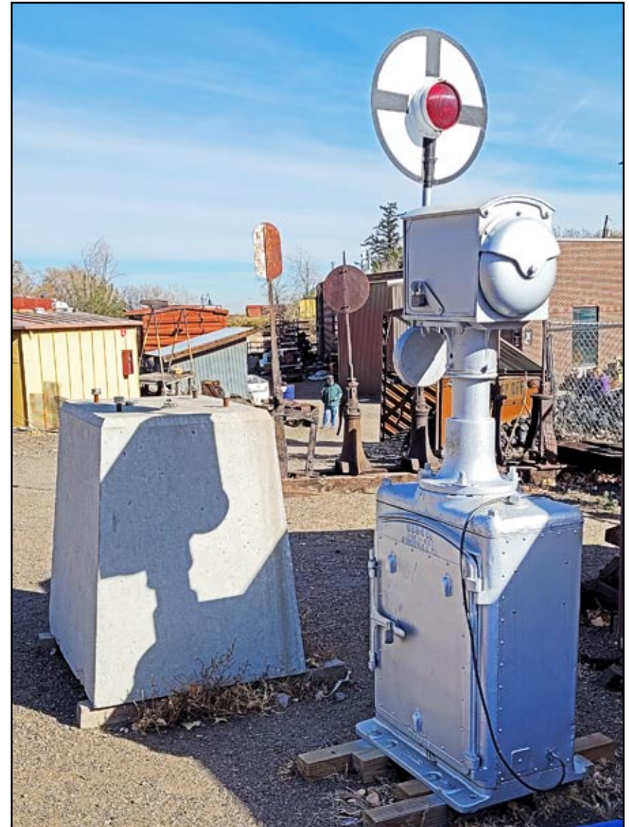
This wig-wag road crossing signal was the last one operating in the state of Colorado. It had been on the old Santa Fe line between La Junta and Trinidad at Delhi until about a year ago. The BNSF retired it, sent it to their signal shop for refurbishment, and then gifted it to the Colorado RR Museum. It should soon be placed on display and in operational condition. Past president Dave Schaaf had a small part in getting it donated to the museum. – Photo © 2022 Dave Schaaf.
